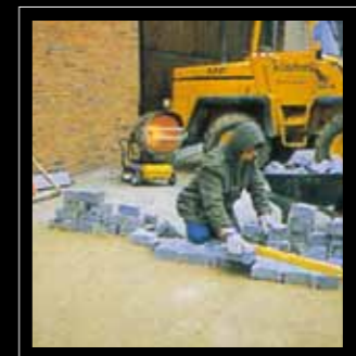
Winter construction: heats up materials, machines, and working sites
